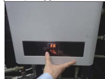
4. Tap on/off icon to enter to FA Tap the on/off icon, when it displays digits. Select the corresponding gas source code.
